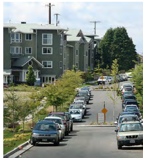
The streets in Seattle's High Point neighborhood help manage stormwater in a number of ways: narrower streets, landscaped buffers with bioswales and street trees, and permeable concrete sidewalks.
