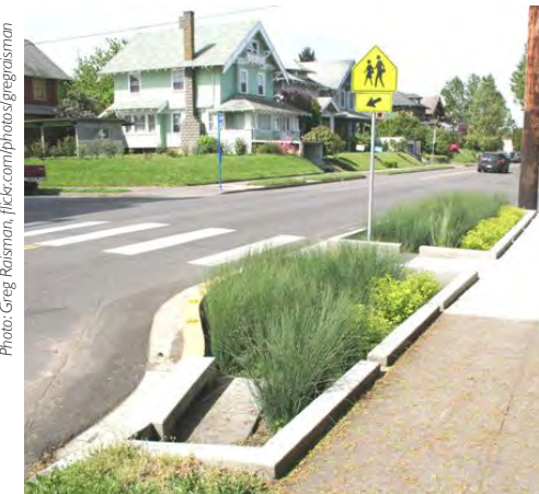
A curb extension in Portland, Oregon provided opportunity to better manage stormwater through a vegetated swale.
