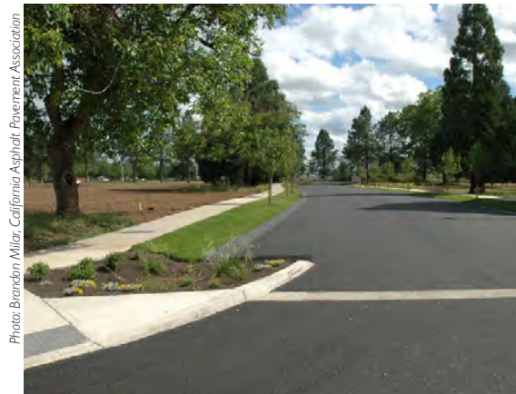
Porous asphalt application in California.
